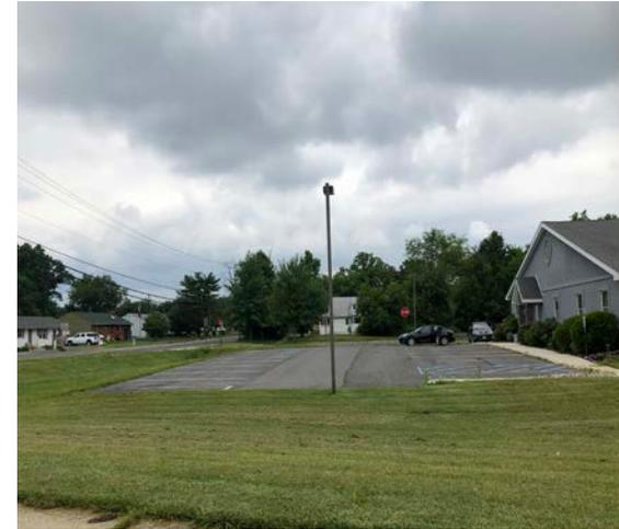
An existing detention basin at the west side of the property can be converted to a rain garden to increase treatment and infiltration of stormwater at the site. Porous pavement can be installed in the parking spaces at the north to capture runoff from the pavement. A preliminary soil assessment suggests that the soils have suitable drainage characteristics for green infrastructure.
