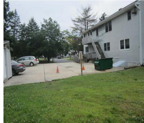
A rain garden can be installed on the southeast side of the building in the turfgrass area pictured above to capture runoff from the impervious roof via downspouts. A preliminary soil assessment suggests that the soils have suitable drainage characteristics for green infrastructure.
