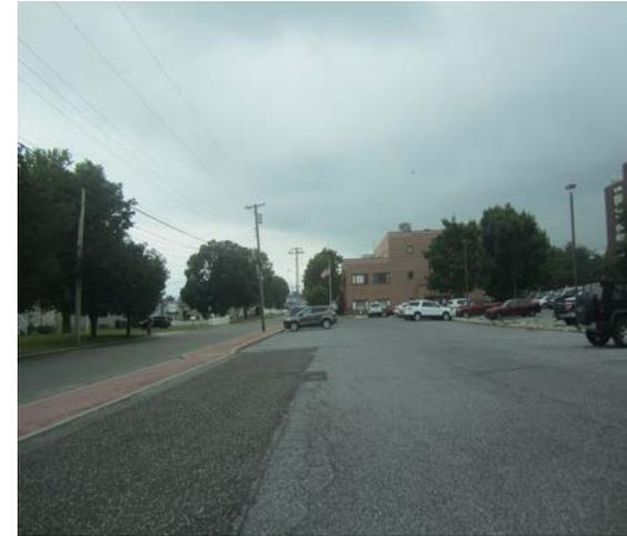
Two sections of parking spaces can be replaced with porous asphalt to capture and infiltrate stormwater runoff from the parking lot. A preliminary soil assessment suggests that the soils have suitable drainage characteristics for green infrastructure.
