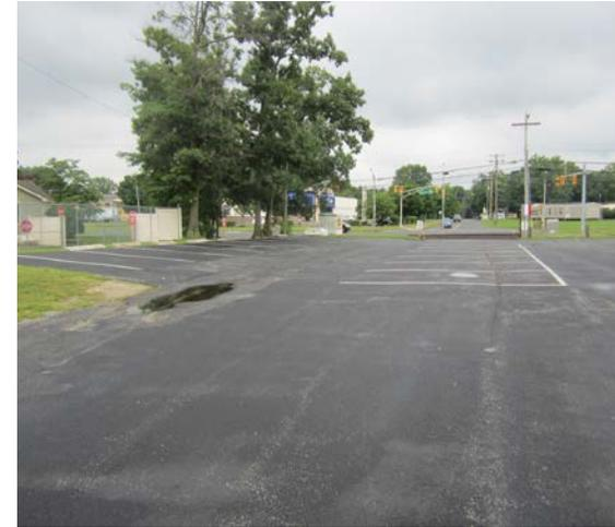
Two sections of parking spaces can be converted to pervious pavement to capture and infiltrate stormwater runoff from the parking lot. A preliminary soil assessment suggests that the soils have suitable drainage characteristics for green infrastructure.
