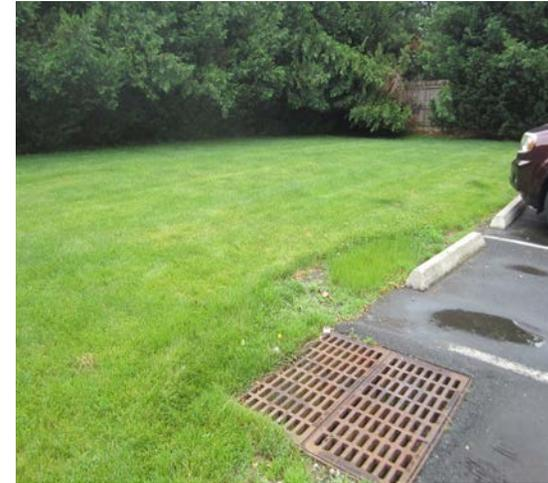
Porous pavement can be installed in parking spaces to capture runoff from the parking lot before entering the catch basin. A preliminary soil assessment suggests that the soils have suitable drainage characteristics for green infrastructure.
