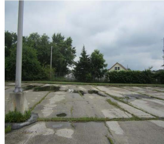
A rain garden can be installed in the turfgrass area near the parking lot entrance west of the building to capture runoff from the impervious parking lot. Porous pavement could be installed in the parking lot in the back toward the northwest of the building to reduce existing pooling and erosion. A preliminary soil assessment suggests that the soils have suitable drainage characteristics for green infrastructure.
