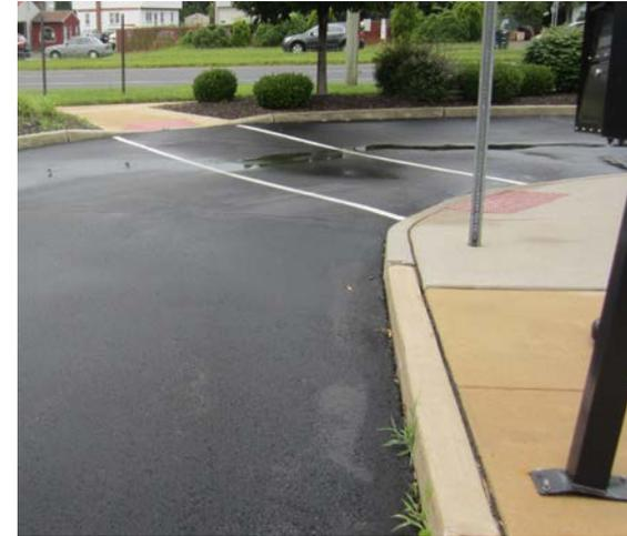
Parking spaces in the parking lot to the southeast of the building can be converted to porous pavement to capture and infiltrate stormwater runoff from the parking lot. A preliminary soil assessment suggests that the soils have suitable drainage characteristics for green infrastructure.
