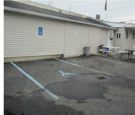
Porous pavement can be installed in the handicap parking spaces next to the building to capture runoff from the roof before entering the nearby catch basin. A preliminary soil assessment suggests that the soils have suitable drainage characteristics for green infrastructure.
